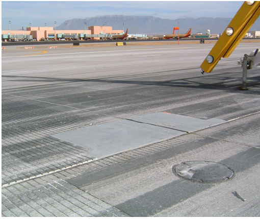
Delpatch™ runway spall repair, Albuquerque International Sunport, New Mexico
