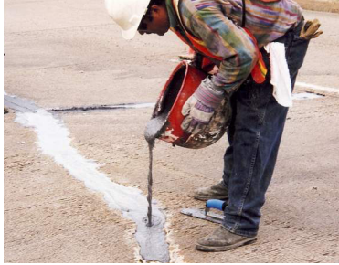
Spall and crack repair, Highway 6, Houston, Texas
