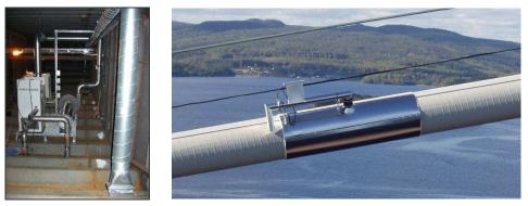
Figure 8 Dehumidification plant and exhaust sleeve
