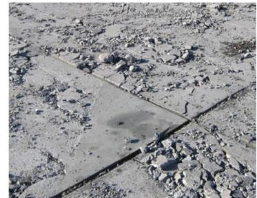
Delpatch repair after being struck by the breaker
