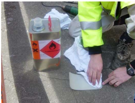
FIGURE 31 CLEAN PATCH WITH XYLENE
