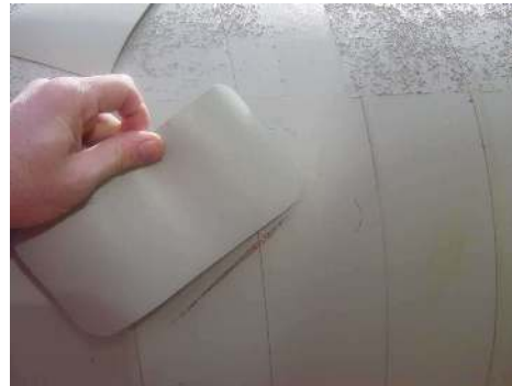
FIGURE 30 PATCH 100MM LONGER THAN CUT
