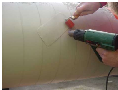
FIGURE 33 APPLY THE PATCH USING A HEAT GUN AND ROLLER
