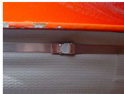
FIGURE 22 STRAP INSTALLED BEHIND INDICATOR BUMP
