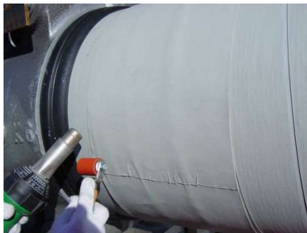
FIGURE 19 HEATING FINISH STRIP
