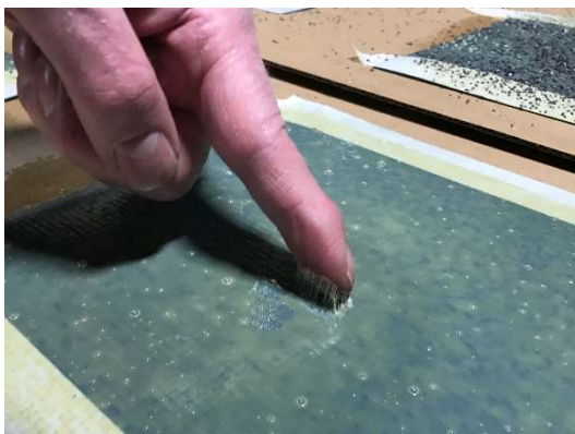
FIGURE 26 45-1 BASE COAT LIFTING & NOT READY FOR TOP COAT APPLICATION
