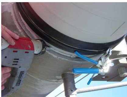
FIGURE 13 APPLYING CAULK
