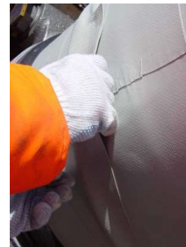
FIGURE 20 FINISH STRIP PULLED BACK
