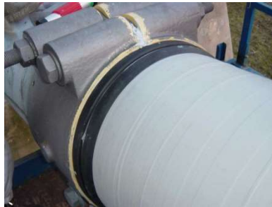
FIGURE 7 WEDGE INSTALLATION
