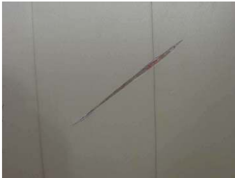
FIGURE 29 CUT LESS THAN 75MM LONG
