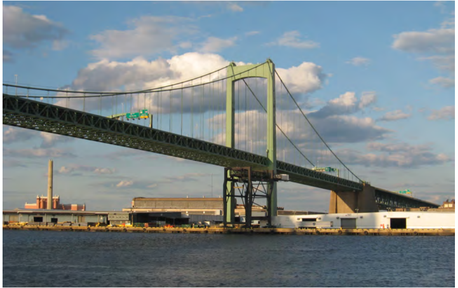
Walt Whitman Bridge, Philadelphia, PA - Versiflex™ Elastomeric Bearing Assemblies.
