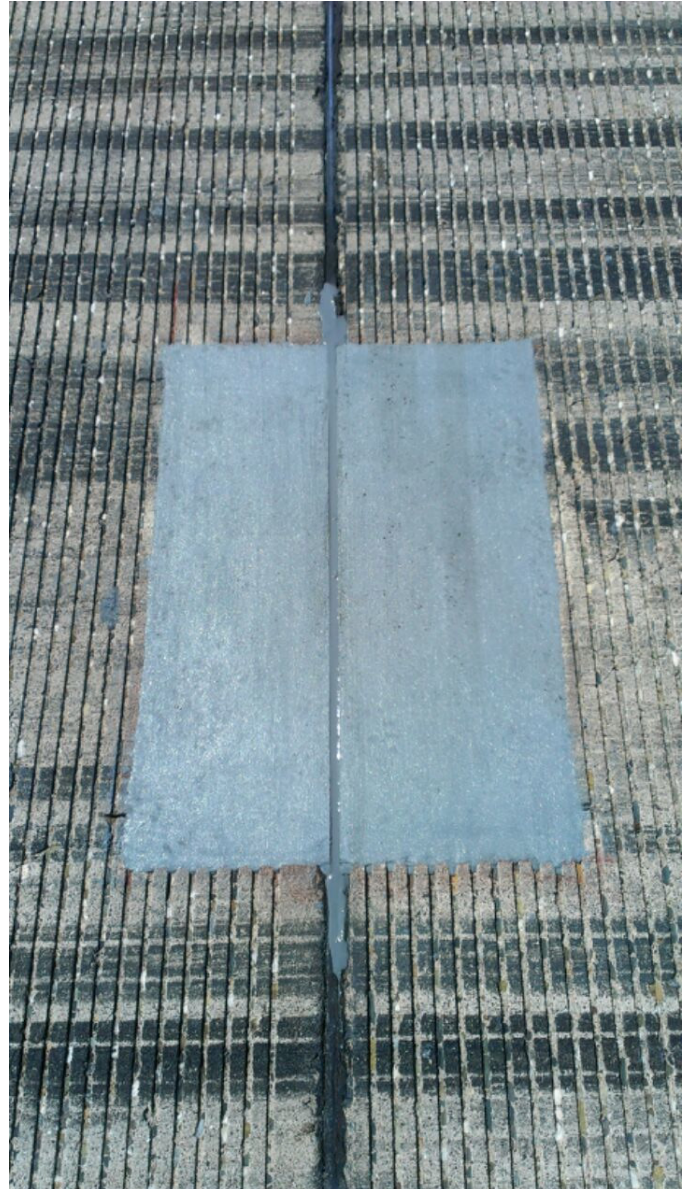
Within an hour, Delpatch™ was ready for airfield traffic.
