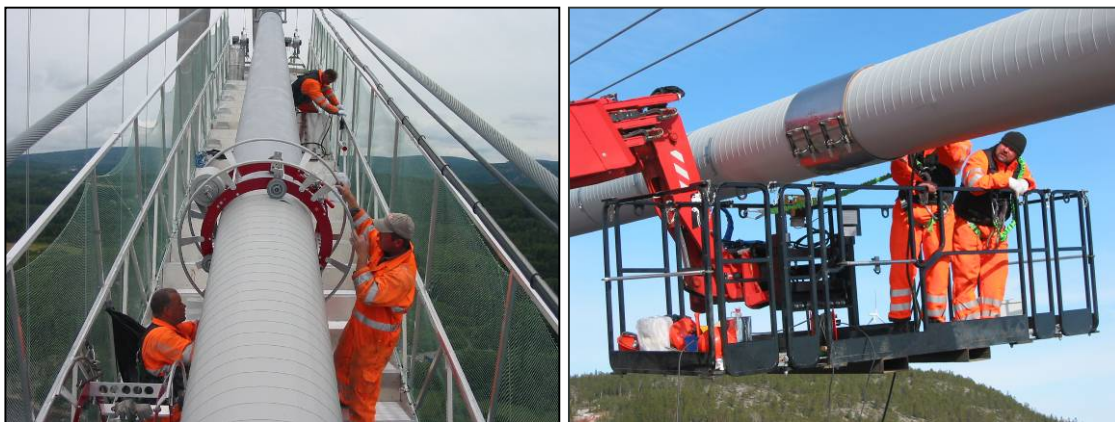
Figure 3 Wrapping and heat bonding of the two layers
