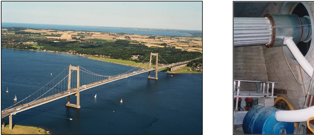
Figure 9 Little Belt Bridge, Overview and on-site injection and flow test
