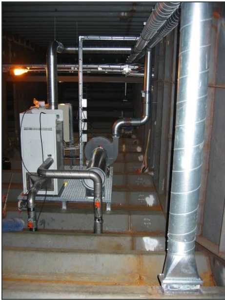
Figure 5 Dehumidification plant (left), injection (upper) and exhaust points (lower)
