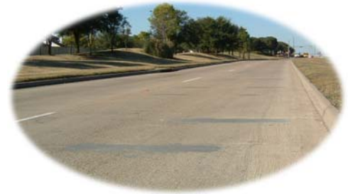
Highway 99 Fort Bend County, Texas
