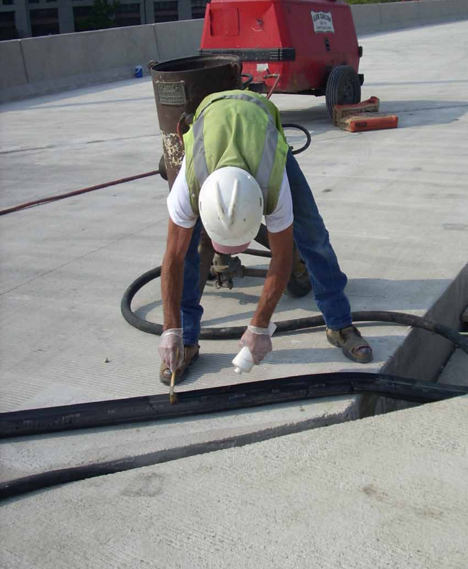
Applying seal conditioner into the ribs of the profile.
