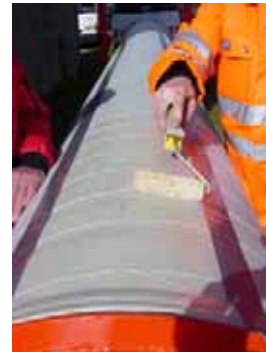
Figure 27 Brush On Base Coat
