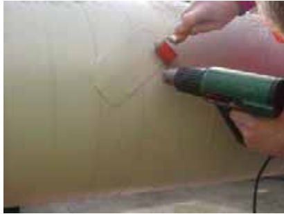
Figure 36 Apply the Patch Using a Heat Gun and Roller
