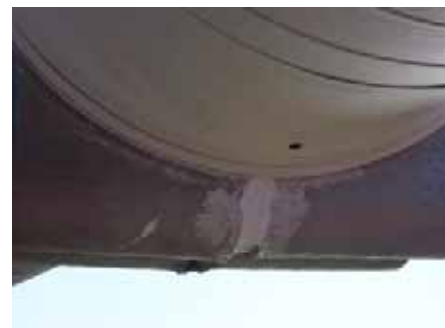
Figure 25 Optional 10mm Hole In the 6 O'clock Position on the Lower Cable Band
