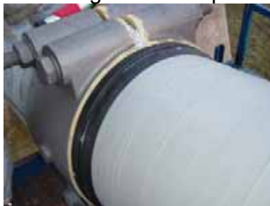
Figure 7 Wedge Installation
