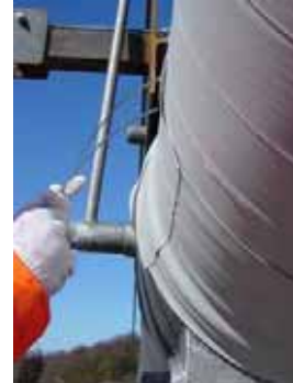
Figure 22 Finished Strip Snapped Over Wedge
