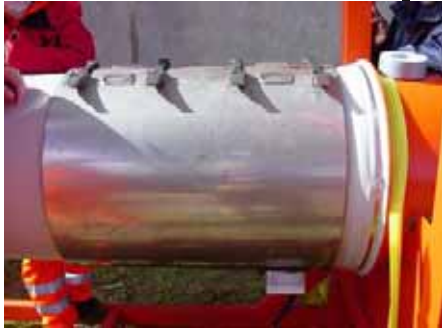
Figure 19 Heating Finish Strip With a Blanket
