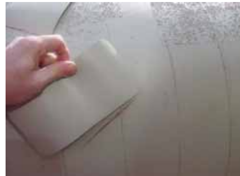
Figure 33 Patch 100mm Longer Than the Cut
