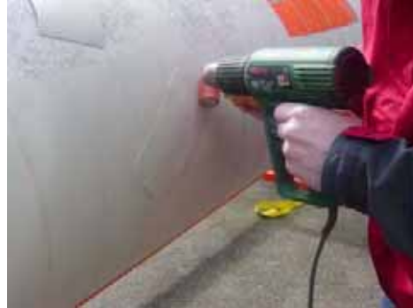
Figure 43 Apply Patch Using a Heat Gun and Roller
