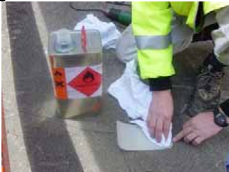
Figure 34 Clean Patch with Xylene
