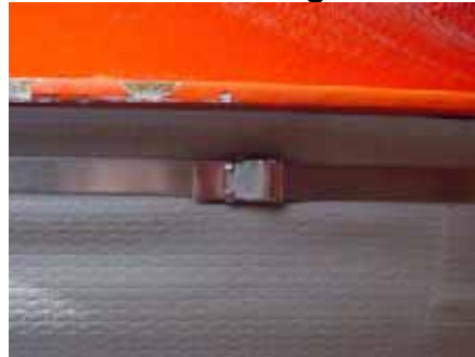
Figure 23 Strap Installed Behind Indicator Bump
