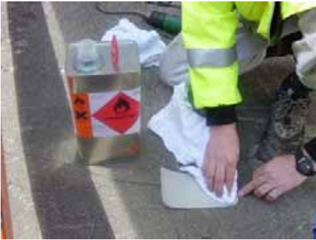
Figure 41 Clean Patch With Xylene
