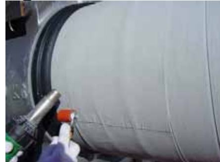
Figure 20 Heating Finish Strip
