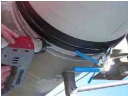
Figure 13 Applying Caulk
