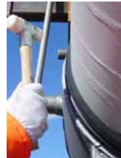
Figure 14 Sliding Wedge Into Place
