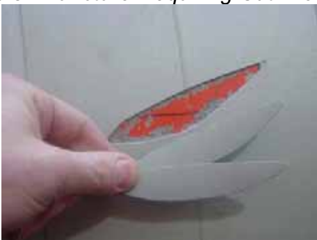
Figure 39 Cut 2 Ply Filler Patch to Match Tear
