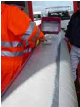
Figure 28 Paint Walk Surface
