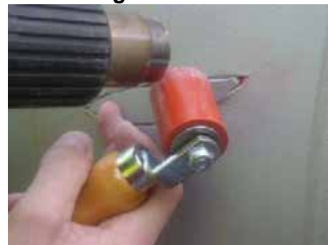
Figure 40 Apply Filler Patch With A Heat Gun and Roller
