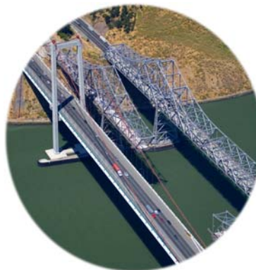
Alfred Zampa Memorial Bridge, California
