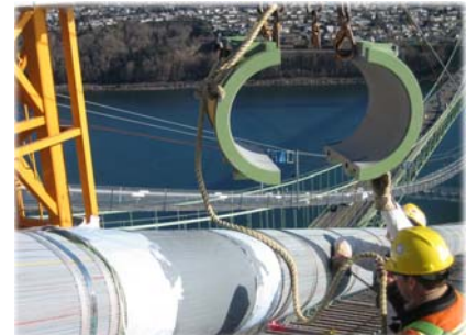
Tacoma Narrows Bridge, Washington State
